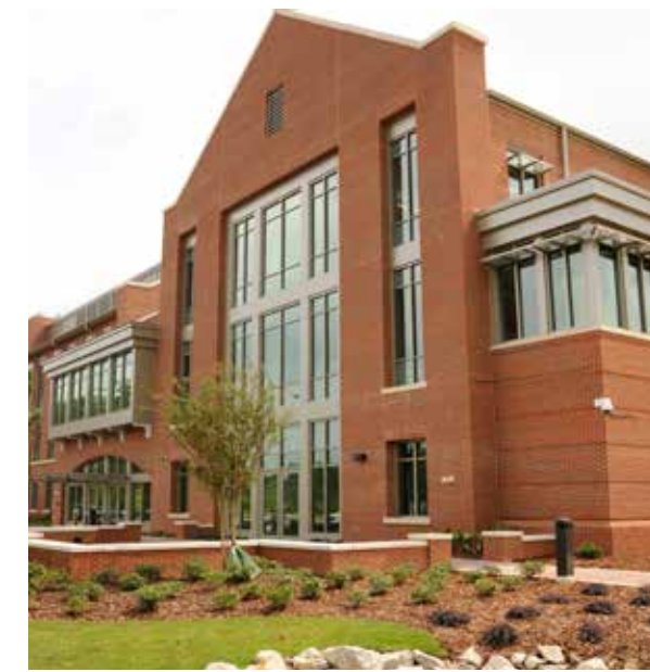
RESEARCH HUB The newly completed 84,000-square-foot Mike Hubbard Center for Advanced Science, Innovation and Commerce is located in the Auburn Research Park off South College Street. The center has the potential to bring in millions of dollars in research grants and contracts annually, which can result in several times that amount in amplified economic impact per year.
